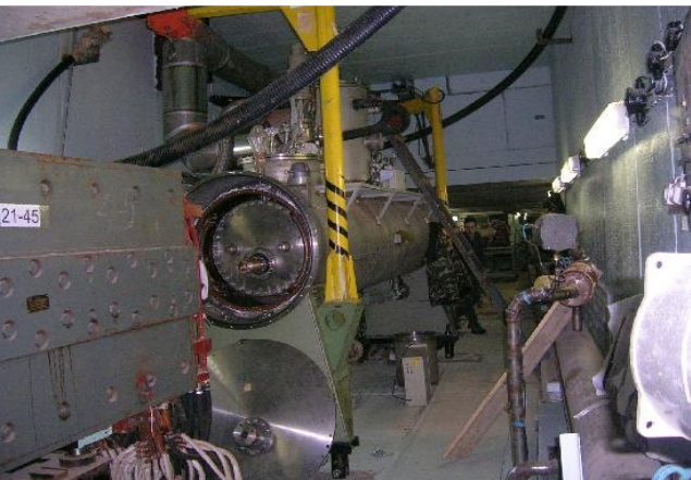
RF deflector in the beam line
